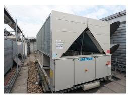
Two Daikin 560kW air-cooled screw chillers were installed to replace the old units,
